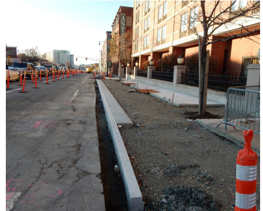
Construction photo of the sidewalk-level separated bike lane on the north side of Route 28 near Water Street (Image looking north west)
