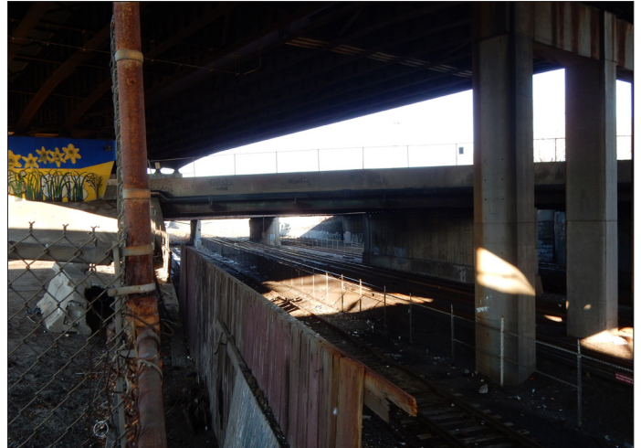
Interstate 93 passes by above Route 38 which travels over over rail tracks. The multiple layers of transportation infrastructure result in difficulty for pedestrians and bicyclists navigating to and through the neighborhood. Image looking north from Brighton Street.
