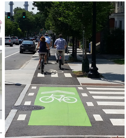
Example of a one-way separated bike lane at sidewalk grade in Cambridge
