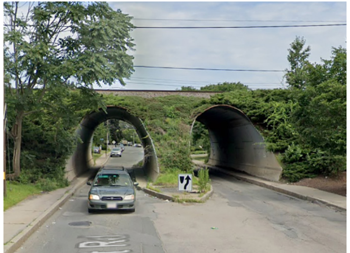
B9: Proposed speed humps, stencils, and a replacement overpass in the long term will improve access and comfort through the existing culverts (Image: Google streetview)
