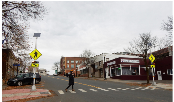
Example of an Rectangular Rapid Flashing Beacon in Greenfield, MA
