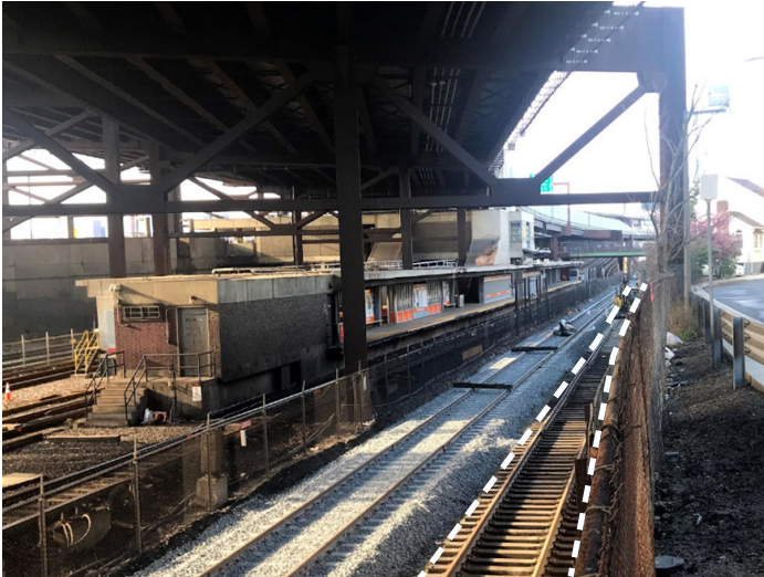
B1: Much of the recommended shared-use path will replace the freight storage tracks on the west (right) side of the ROW. (Image: Deniz Karakoyunlu.)
