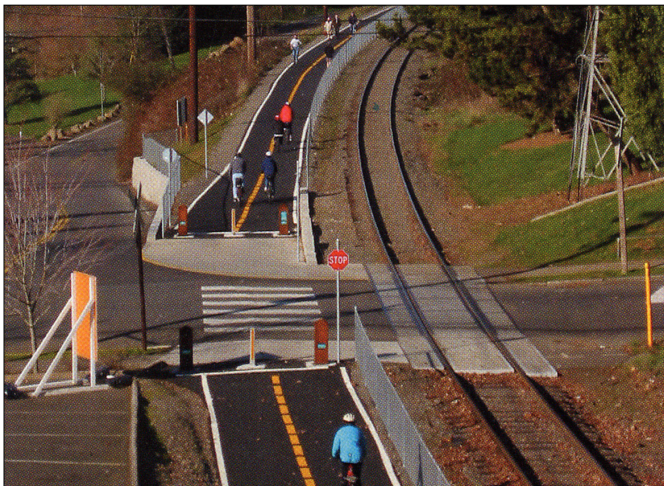
The Springwater Corridor Trail in Portland OR features a 10' setback from the centerline of the tracks
