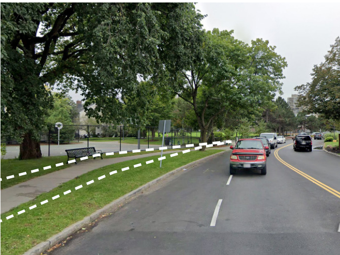
A3: The sidewalk on the south side of Rufo Road can be widened to accommodate a shared-use path
