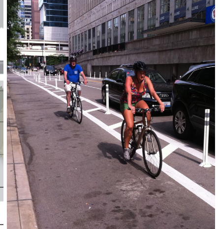
Example of a one-way separated bike lane adjacent to a sidewalk in Chicago
