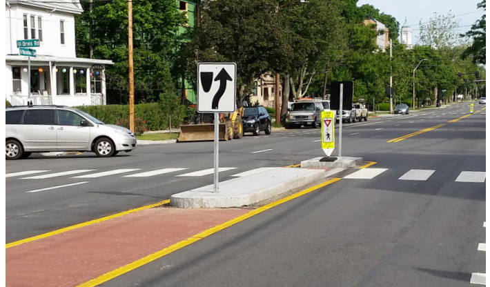
Example of a median refuge island on Massachusetts Ave. in Arlington, MA
