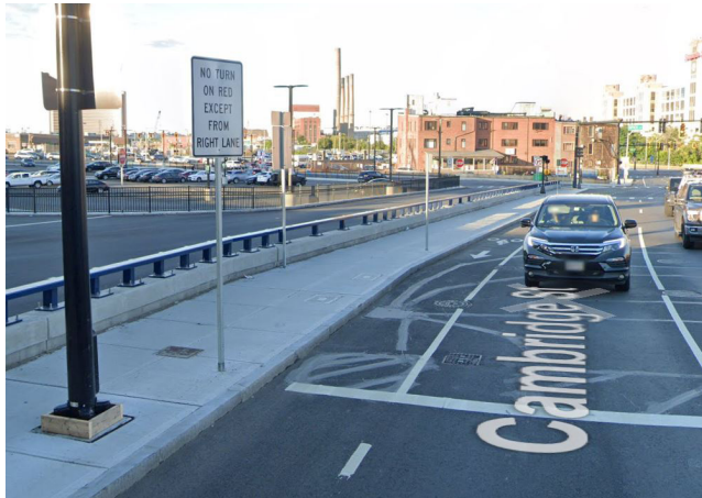
On the east side of the I-93 overpass, the proposed route would widen the existing sidewalk to accommodate a barrier-protected shared-use path, which would require removal of the existing on-road bike lane. (View looking east. Image: Google street view.)
