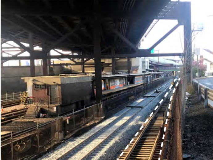
B1: Much of the recommended shared-use path will replace the freight storage tracks on the west (right) side of the ROW. (Image: Deniz Karakoyunlu.)
