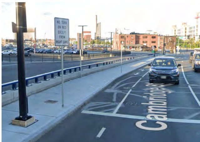
On the east side of the I-93 overpass, the proposed route would widen the existing sidewalk to accommodate a barrier-protected shared-use path, which would require removal of the existing on-road bike lane. (View looking east. Image: Google street view.)
