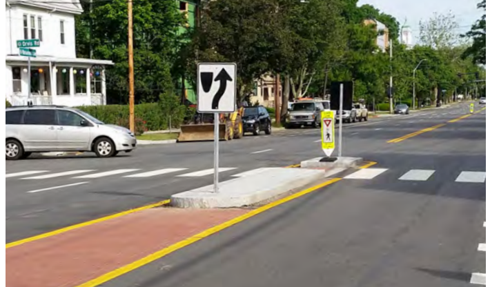
Example of a median refuge island on Massachusetts Ave. in Arlington, MA
