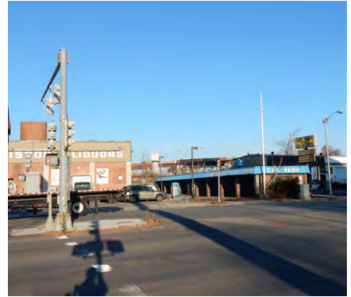
Route A1 (and A2) would provide pedestrian and bicycle infrastructure improvements at the Rufo Road/McGrath Highway intersection (Image looking north east)
